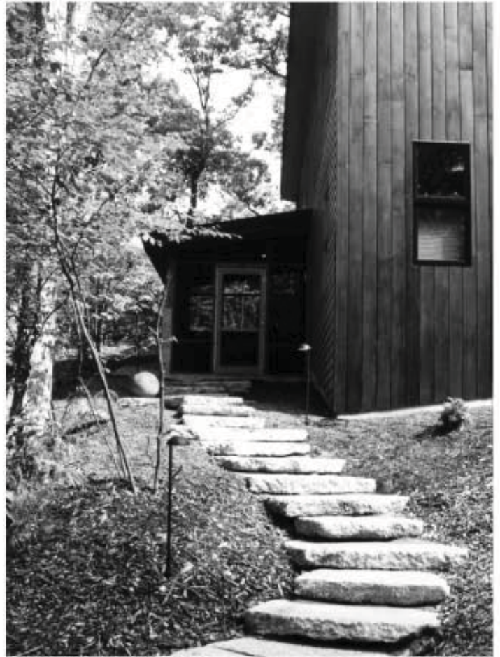
Wood chips blanket the steep dune; the stairway consists of chunks of street pavement salvaged from a vacant lot in Michigan City.
