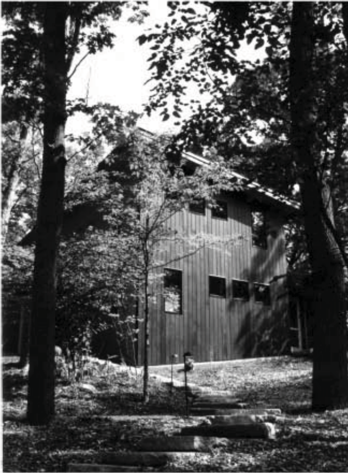
Blending with the tall trees of Shoreland Hills, the house built by Larry Zimmer and Ted Perzanowski was designed to harmonize with nature.
